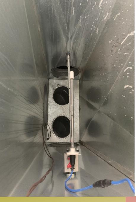
Germicidal Blue Non-Ozone UV Light Tubes were installed in all HVAC units to ensure that indoor facilities have adequate ventilation. These light tubes must be changed every year. They extend the life of the air system by keeping coils and drain pans free of mold and improve indoor air quality by killing airborne bacteria and viruses.
